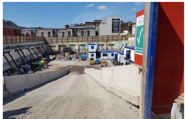
Figure 5 Cleared site of former Odeon complex
